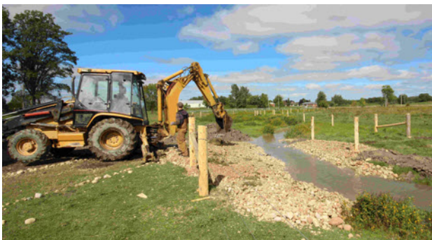
Chub McComb & staff of Black Sheep Fencing install fencing & a farm machinery crossing on Kilsyth Creek (Sept. 2013)
